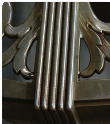
Fixture Before Restoration
