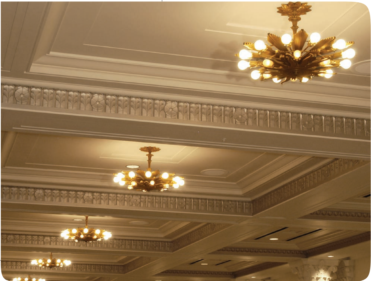
Restored and reinstalled chandeliers
